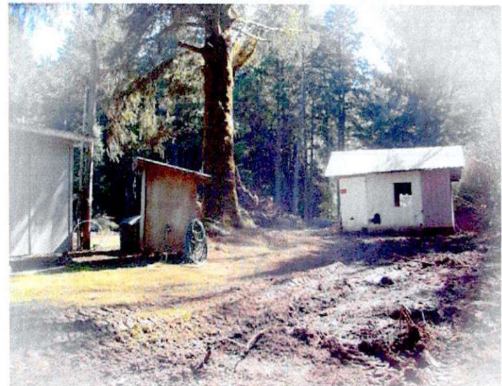
Pumphouse (left) and shed (right) – looking south.
