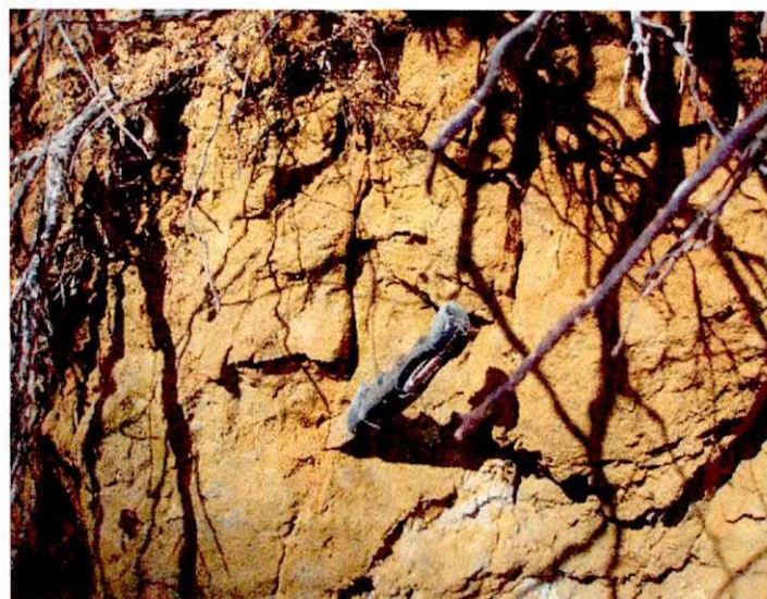
Close-up view of stabilized dune sand comprising the cut bank.
