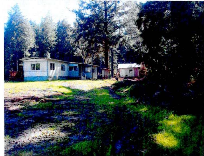
Looking south-southeast from the dug well or cistern. Note wet soil in foreground and soil and slash fill (center right).
