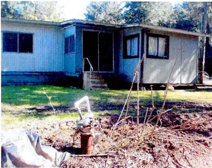
Drilled well with six-inch steel casing west of existing trailer.
