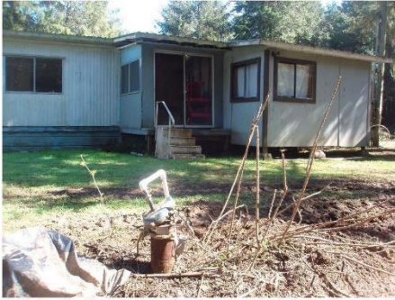
Drilled well with six-inch steel casing west of existing trailer.
