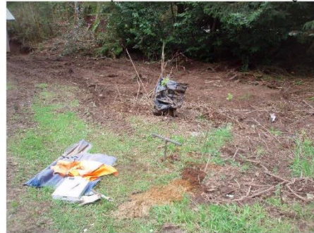
HA2 advanced near drilled well (background) – view southwest.
