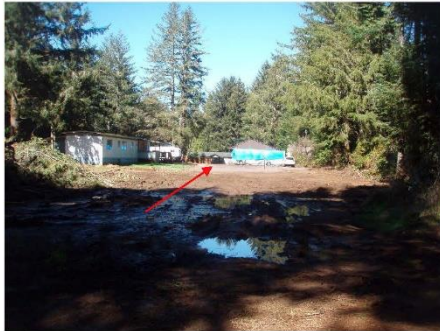
Looking north from the trail in the southern portion of the site at the proposed manufactured home site (center).
