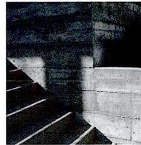
BOARD-FORMED CONCRETE
