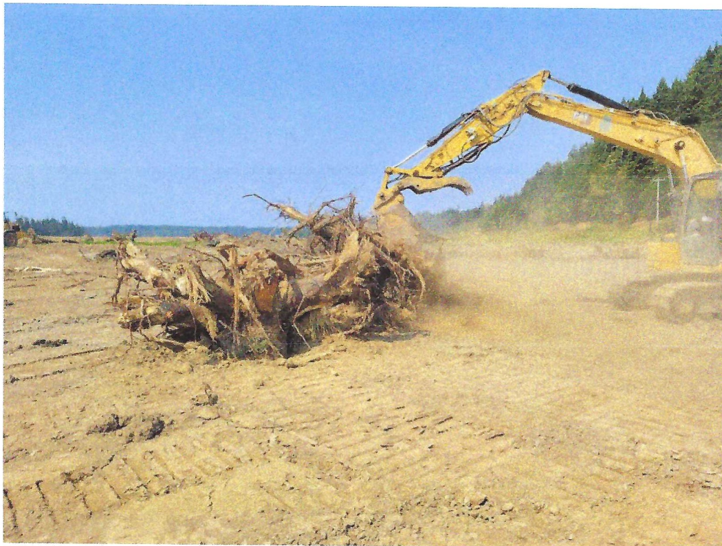
Figure 5. LWD fully installed North Bank Working Landscapes Project, in September 2023.
