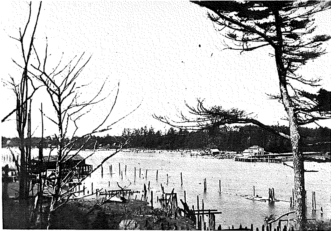
Figure 13. View northwest from the bluff within the current Rogge Mill property, showing the industrial building adjacent to the ferry landing on the left, and the Bullards area on the north.
