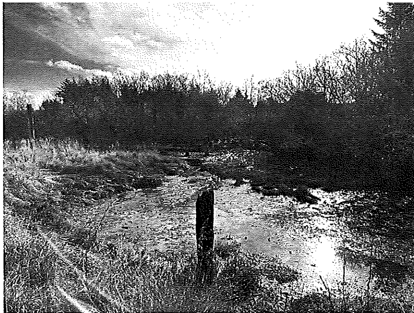
Figure 33. The remains of the boat ramp of the Bullards Ferry south landing, comprised of piers that supported the ramp and at least one horizontal element.
