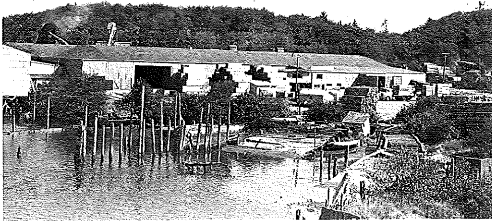
Figure 19. "Rogge Lumber Sales, September 1970." Note the still extant but dilapidating ferry landing ramp, and the adjacent dock to the right, now collapsed. The square concrete structure that once stood on the dock is still extant on the lower right of the picture. The earthen ramp in the right foreground is still extant, and was likely built for the Highway 101 bridge construction.
