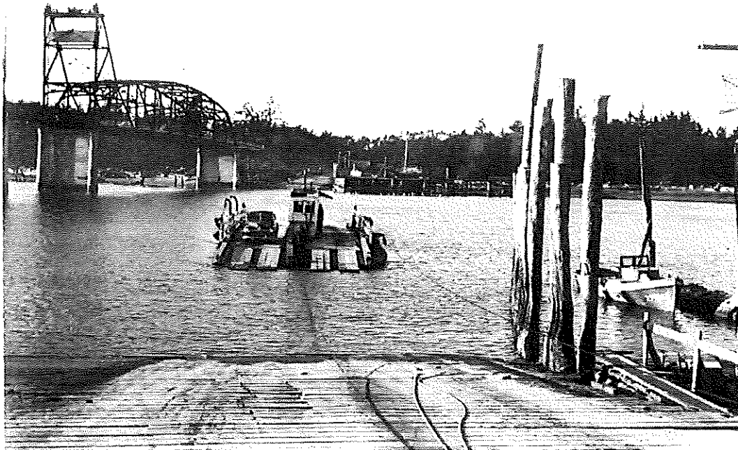
Figure 10. Photograph marked “last trip of the Bullards Ferry, mid-1950s” taken view north from the south ramp within the current project area. (Bandon Historical Museum, photo 30017).
