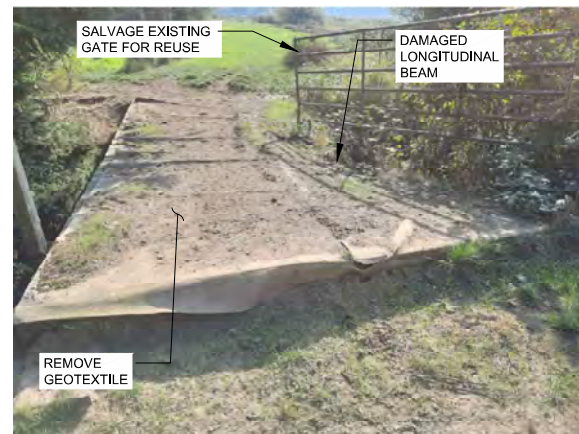
3 EXISTING BRIDGE - LOOKING SOUTH ACROSS BRIDGE Scale: NTS
