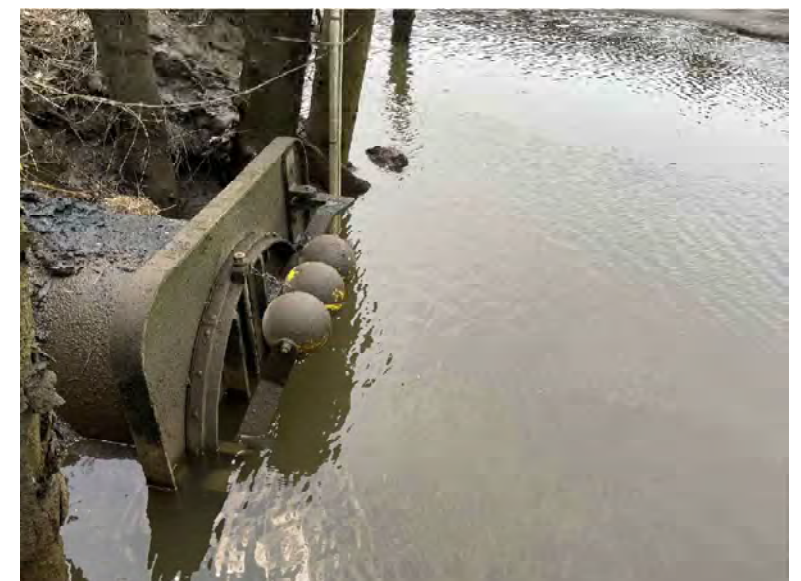
4 SIDE HINGED TIDEGATE WITH MITIGATOR AFTER INSTALLATION Scale: NTS
