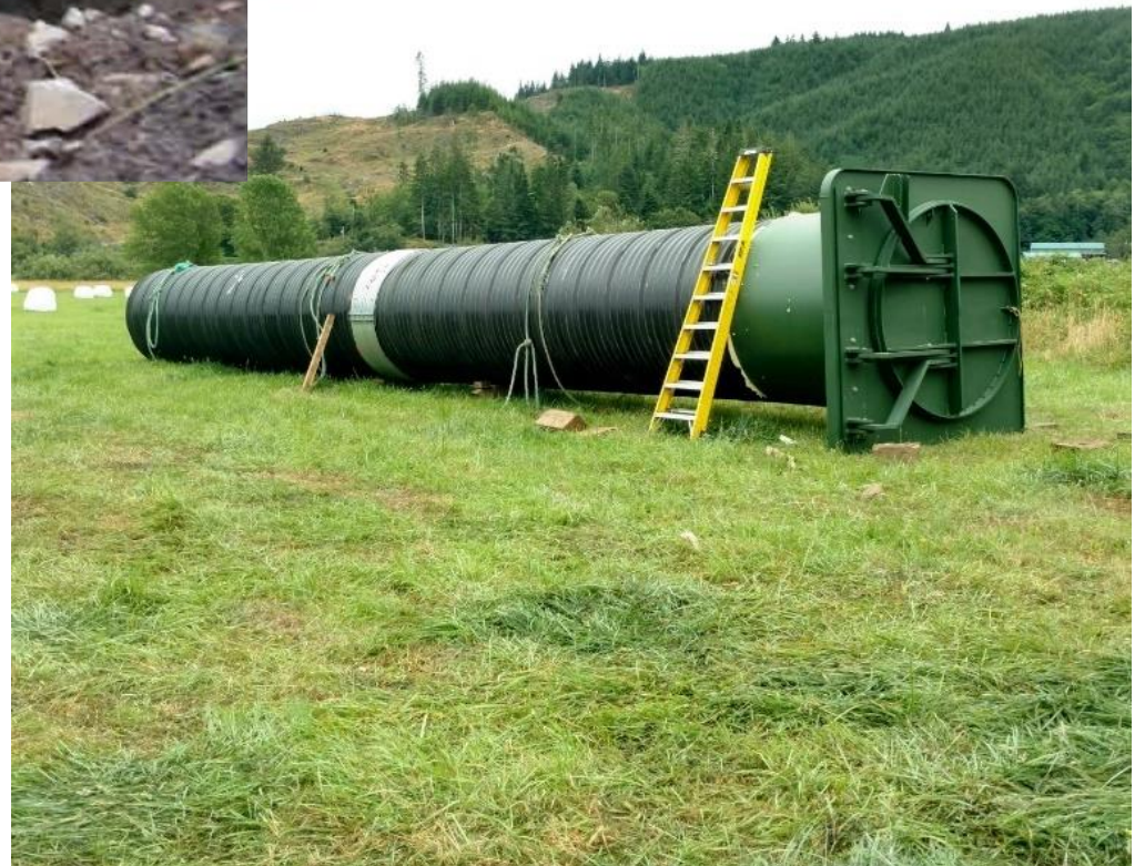
Figure 13. Examples of a side-hinge aluminum tidegate
