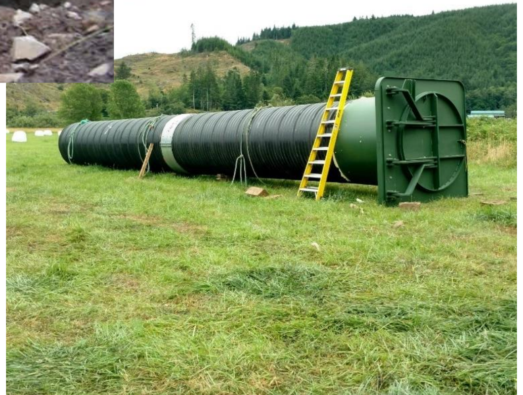
Figure 13. Examples of a side-hinge aluminum tidegate
