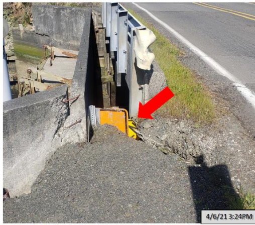
Head wall failure (south side)
