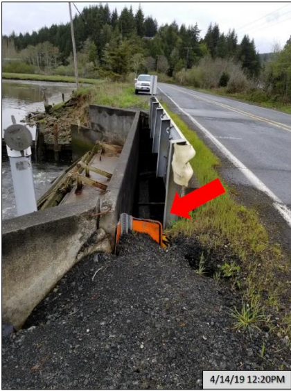
Head wall failure (south side)
