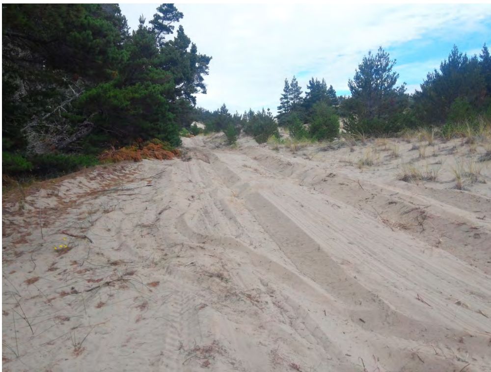
Road cut by bulldozer to help trucks enter area.
