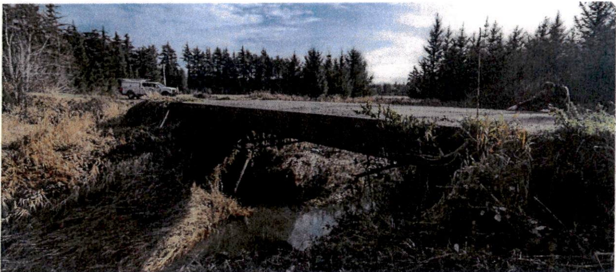
Figure 1. Elevation view of the bridge, looking east
