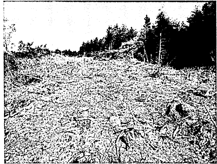
Looking north from southern extent of cleared proposed buildable area.
