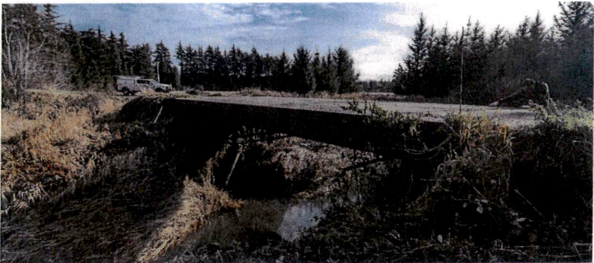
Figure 1. Elevation view of the bridge, looking east
