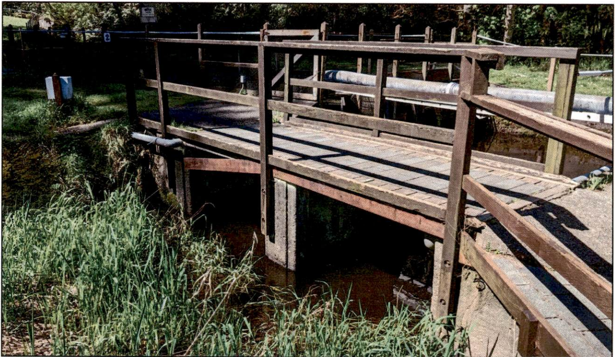
Figure 6. Existing conditions of the upstream footbridge (Station 483.5 ft)
